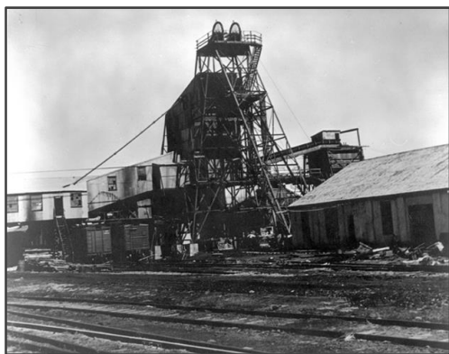
Cadillac Mine, Shaughnessy, Alberta Shaughnessy after 1927 Courtesy Provincial Archives of Alberta: A3465
